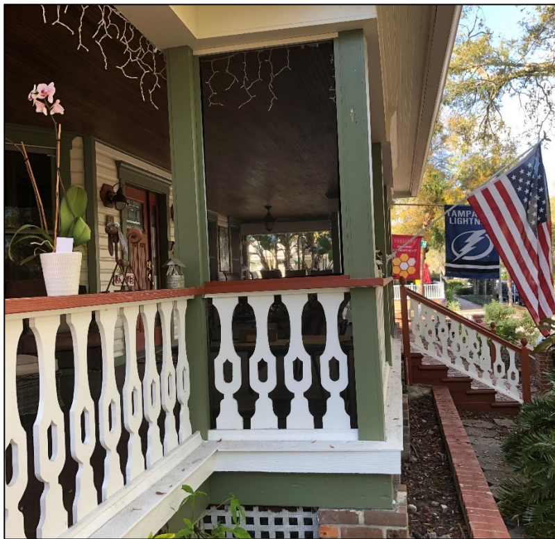
Figure 1: Photograph showing the proposed screen, installed on a portion of the porch.
