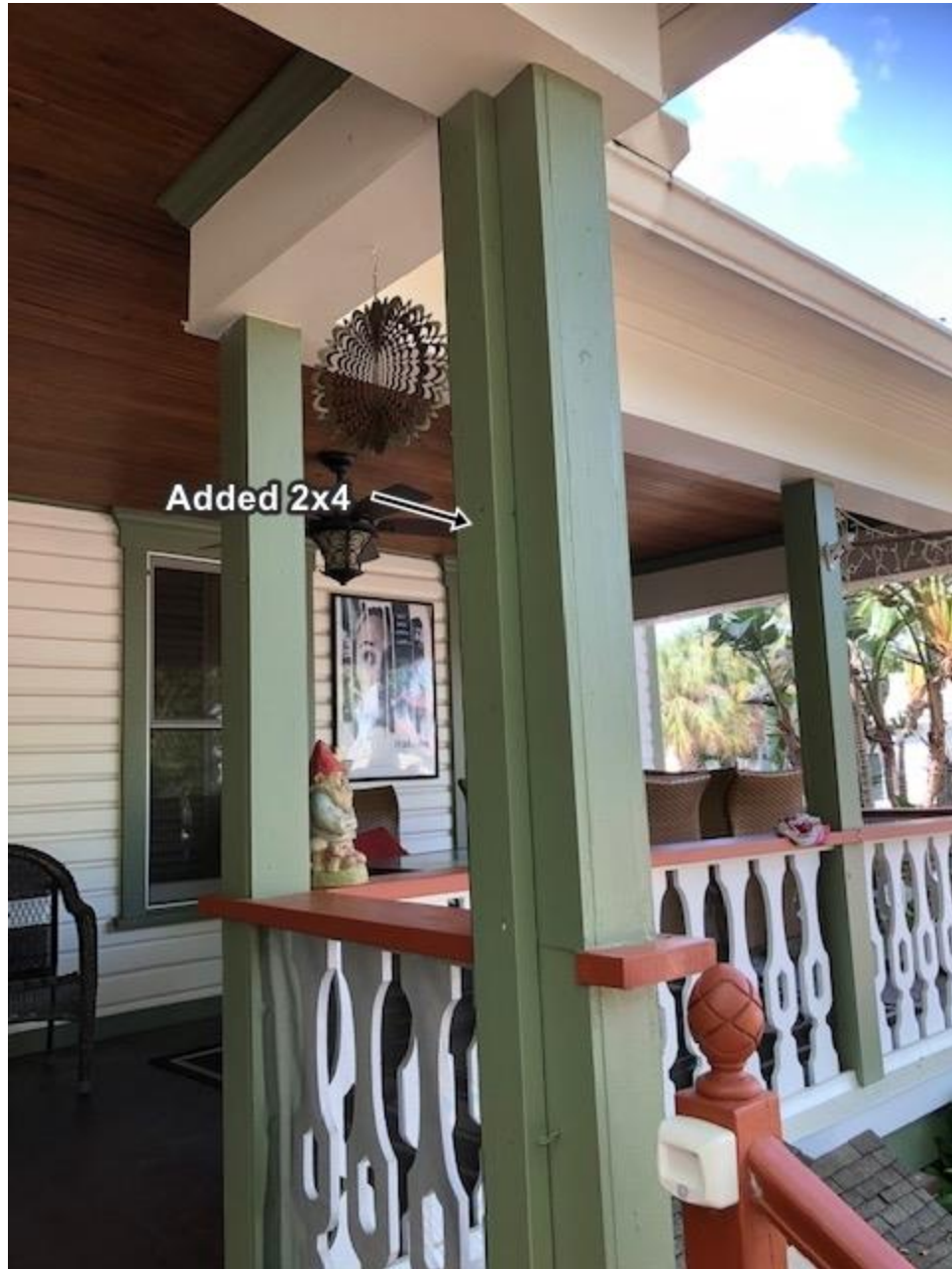
Photo 6 - Right side post with added 2 x 4
