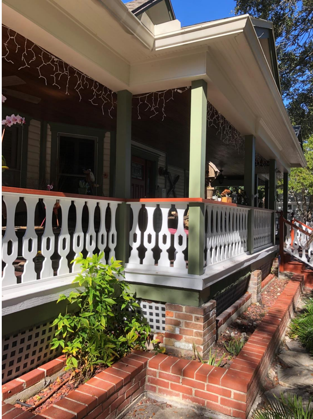
Photo 1 - Side Opening - No molding or screening
