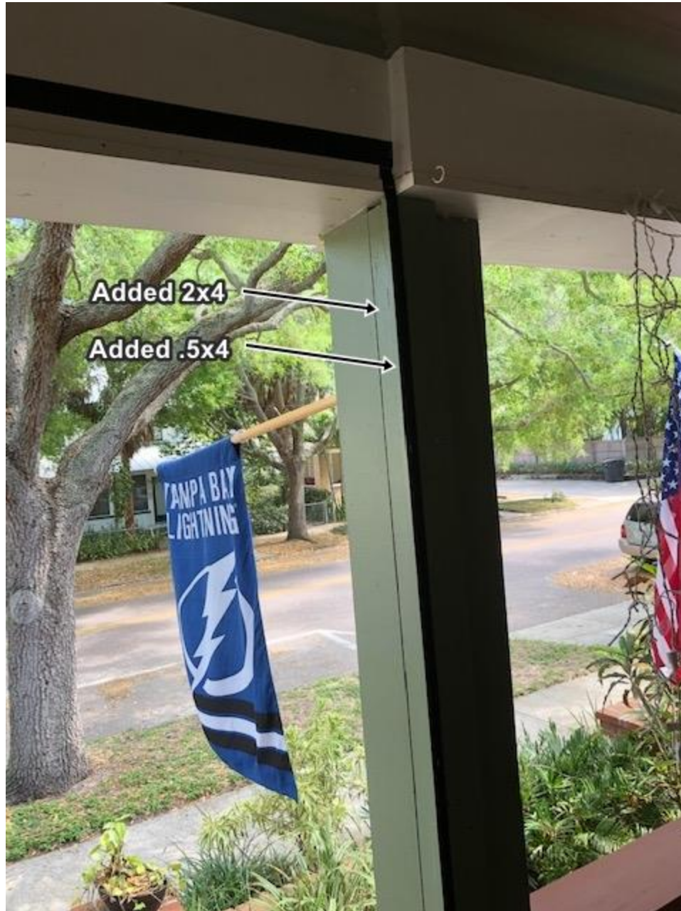
Photo 7 - Left side post with added 2 x 4 and .5 x 4
